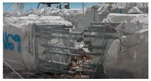
Proximity of reinforcing steel in building and garage columns
