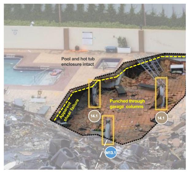
A Pool deck with punch through of columns down to garage
