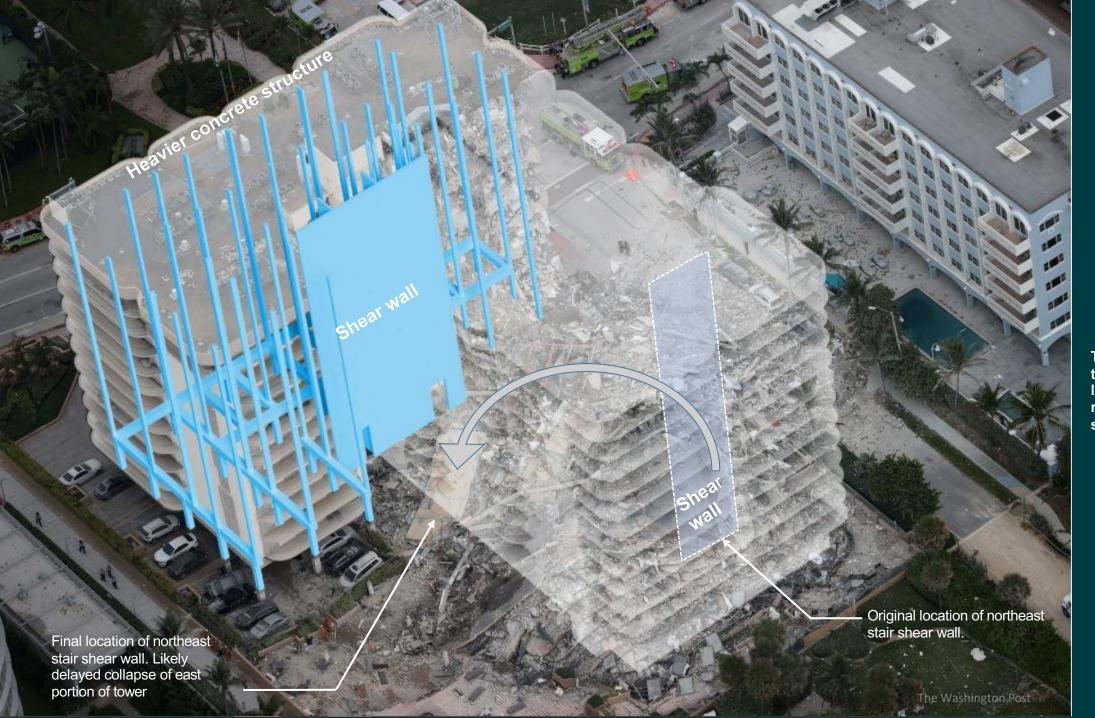
The west portion of the tower remains standing likely due to a more robust structure and sizeable shear wall
