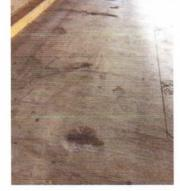
Figure J2: Spalling with exposed steel reinforcement at topside of garage deck.
