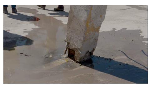
Corrosion of columns at garage slab and foundation
